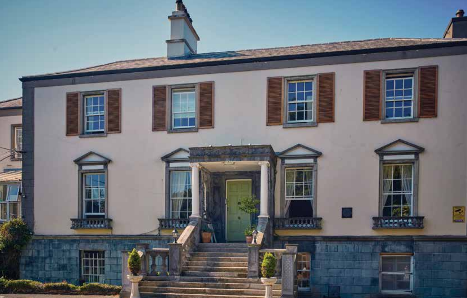
Rutland Centre main house
