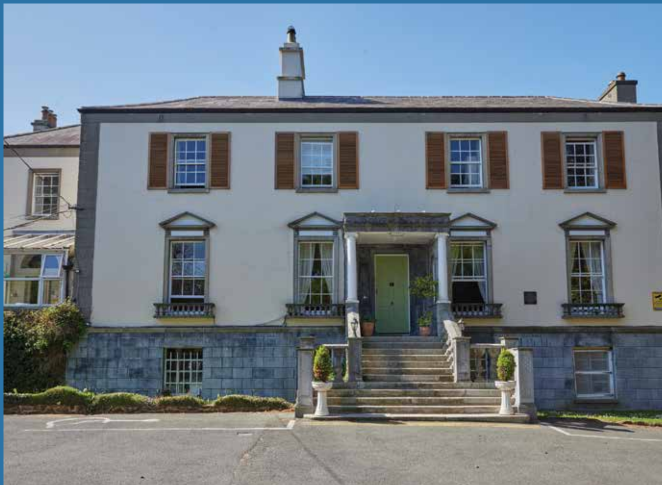
Rutland Centre Main House
